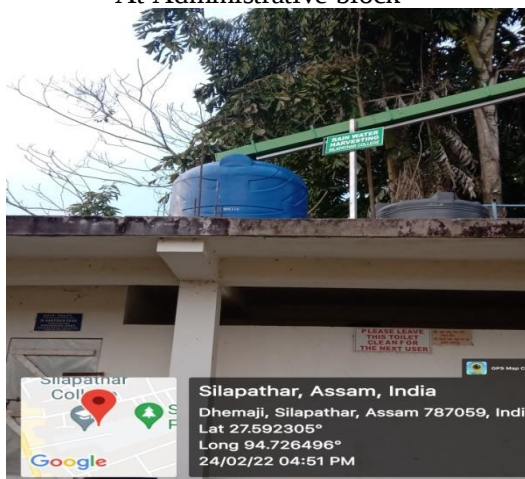
At Students Toilet
